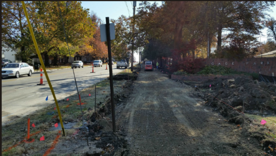
Gage Park Construction at Gage between 6th-10th
