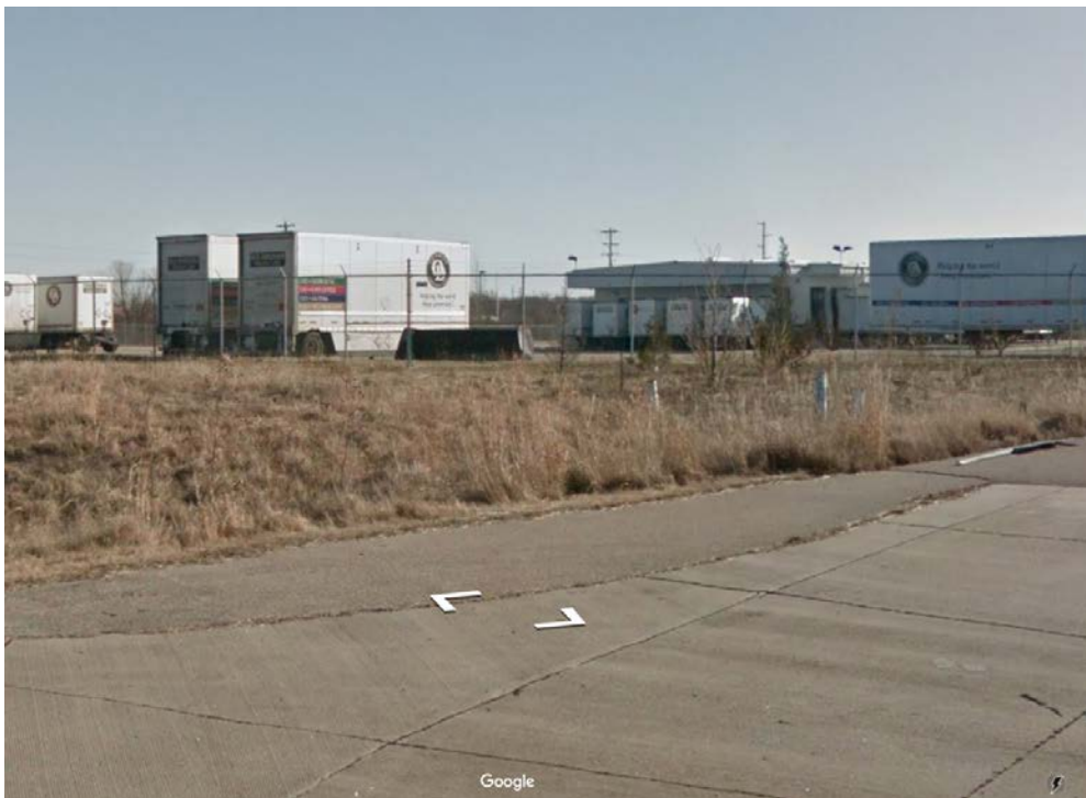
View from SE Cypress Drive (northwest corner)
