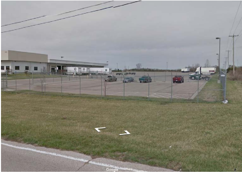
View from SE 21 st Street (southeast corner)
