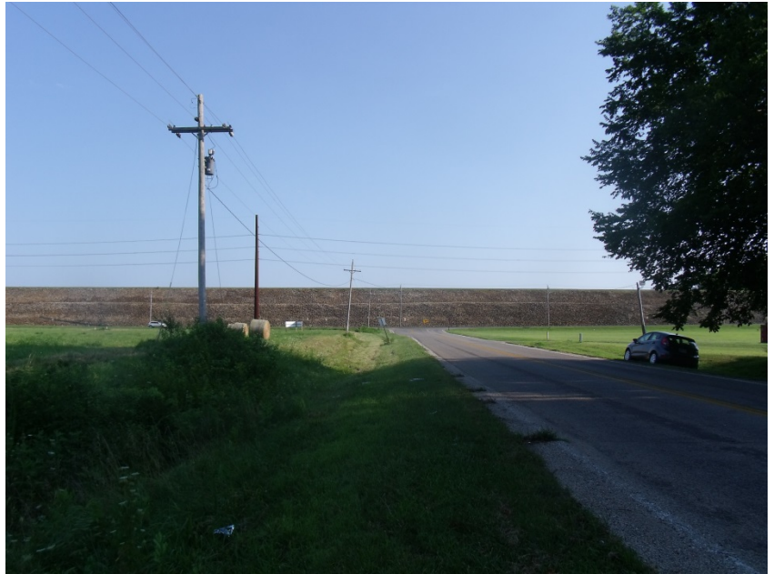
West side of project area looking south along SE Wittenberg Road with Shawnee Lake dam in background
