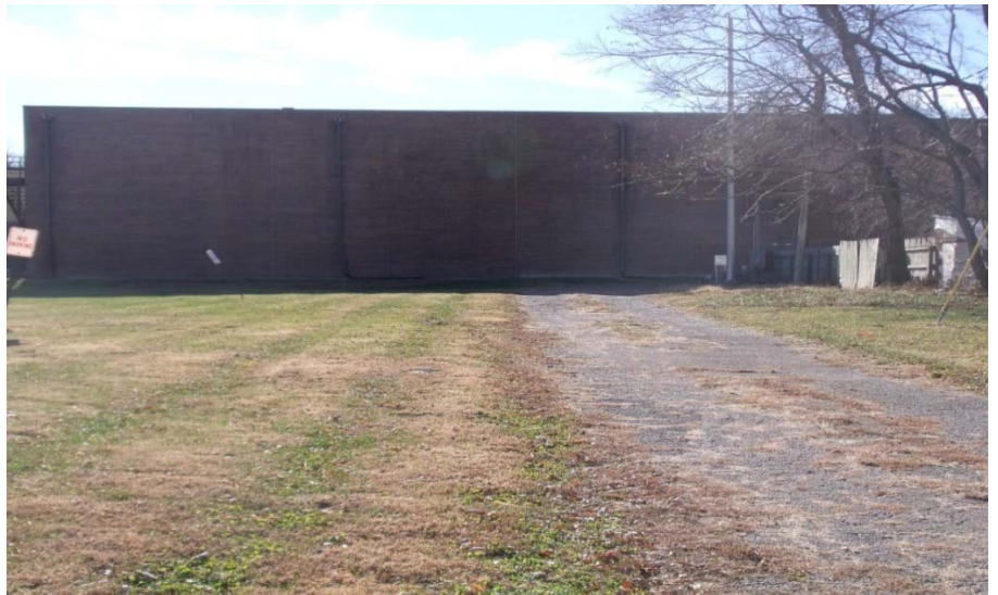
View from south side of Williams Street facing south along access driveway for existing pump station equipment on right, with North Topeka YMCA building beyond.
